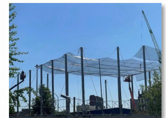
Top: Netting used to protect fans from projectiles can be repurposed to disrupt sUAS flight and observation. Bottom: Anti-drone netting installed to protect critical infrastructure from overhead threats..
